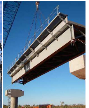
PILBARA RAIL BRIDGES, WA CONTRACT VALUE $8M
