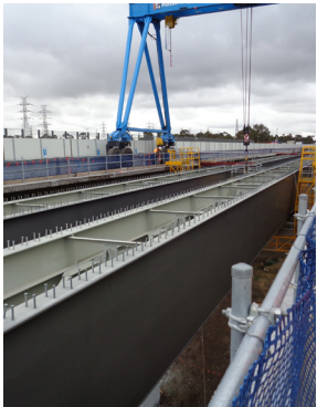
M80 E.J. WHITTEN BRIDGE, MELBOURNE CONTRACT VALUE $9M
