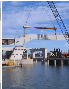
PORT RIVER ROAD & RAIL BRIDGE, PORT ADELAIDE CONTRACT VALUE $12M
