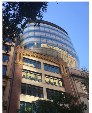
SUB STATION NO.164, SYDNEY CONTRACT VALUE $8M
