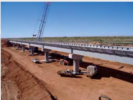
↓ BELOW Rail bridge modules from 43 tonne to 159 tonne, installed on-site in the Pilbara.
