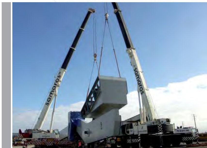
↑ ABOVE Two-crane lift, trial assembly of Port River Rail Bridge.
