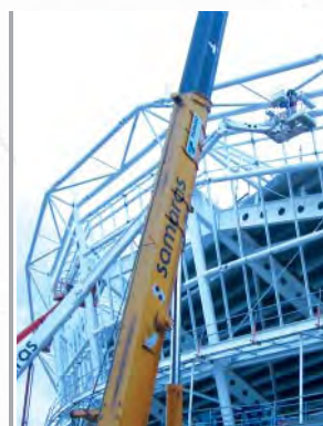
← LEFT Site assembly of the rear glazing structure of the Melbourne Sports & Aquatic Centre.
