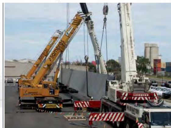
↓ BELOW Four-crane lift, rotating Port River Bridge girder.
